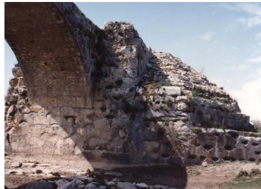
Figure 11. One of the feet of the bridge from the Roman era
