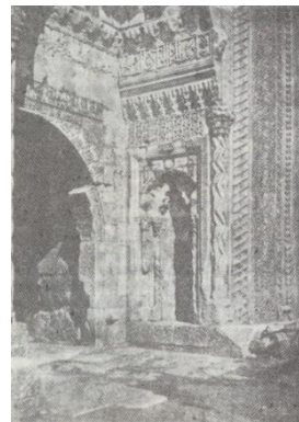
Figure 2. Sultan Han Portal 19 century (Y.Önge's archive)
