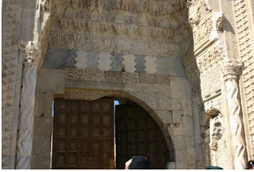
Figure 3. The Flat Camber Arch and The Inscription
