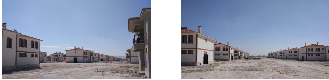
Figure 9. General views inside the construction site of Bozkır Barrage Resettlement Project (Süheyla Büyüksahin's personal archive, August 2020)
