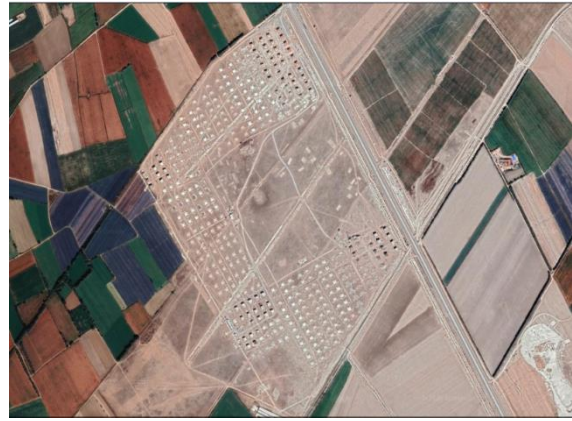
Figure 6. Settlement view of Bozkır Barrage Resettlement Site (google earth, 2020)
